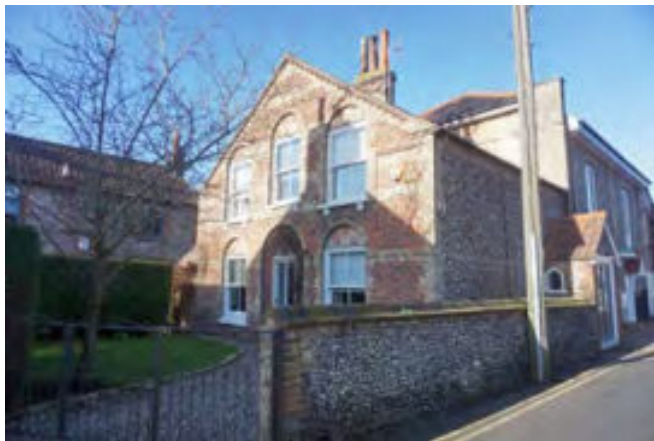
Converted Corn Hall on Albert Street
