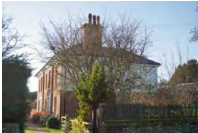
Converted Police Station on Station Road
