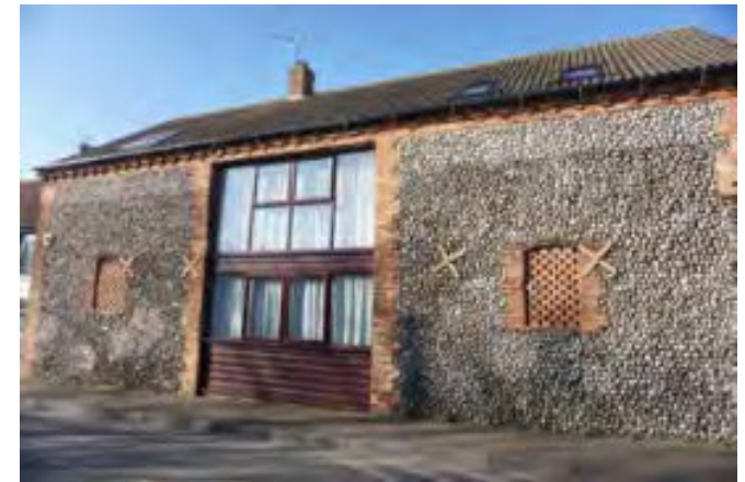
Converted barn on Valley Lane
