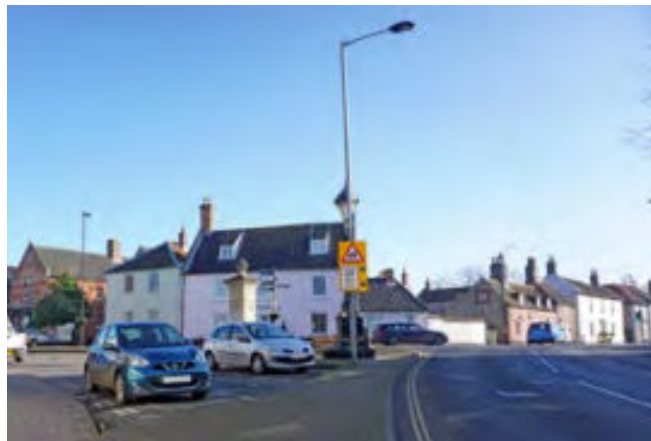
Modern road signage obscuring the Victorian fountain/lamppost
