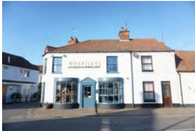
Georgian Shop front with elegant bay windows. Applied lettering to the frontage is a good alternative when a fascia is not available
