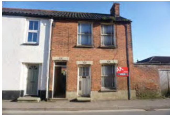
Vacant property on New Street
