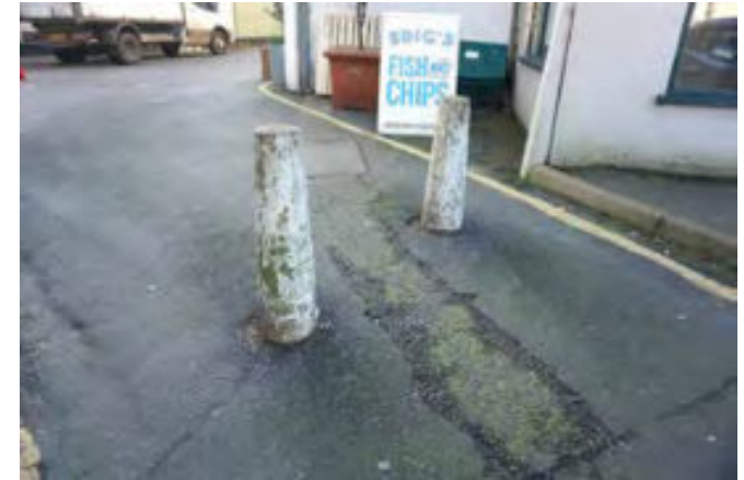
Unattractive concrete bollards with peeling paint
