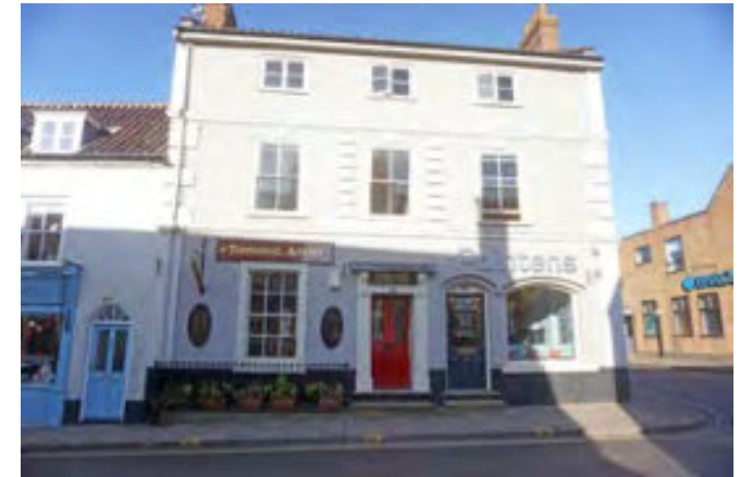
Georgian building on the High Street, with painted brick and large ground floor windows instead of shop fronts
