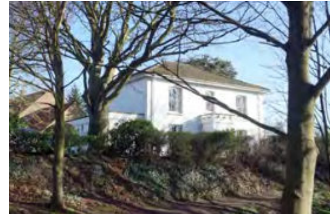
Early-twentieth century house adjacent to the Horn Pits newly included within the Conservation Area boundary (area F on the plan)
