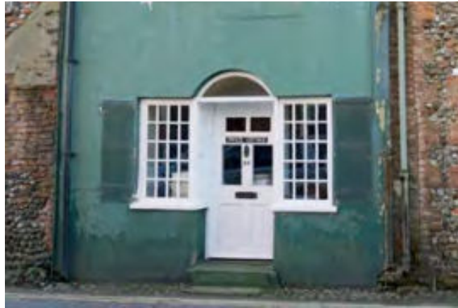
Poor condition of paintwork
