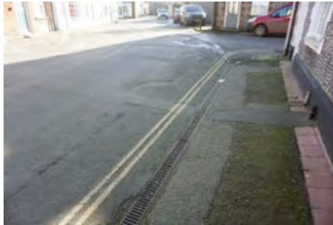
Yellow lines denoting pedestrian walkways where there are no pavements
