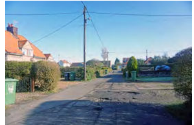
Poor surfacing of The Fairhaven
