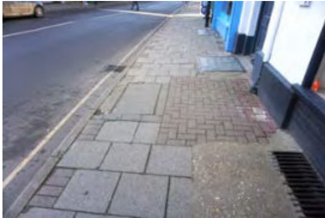
Patchy surfaces on the High Street
