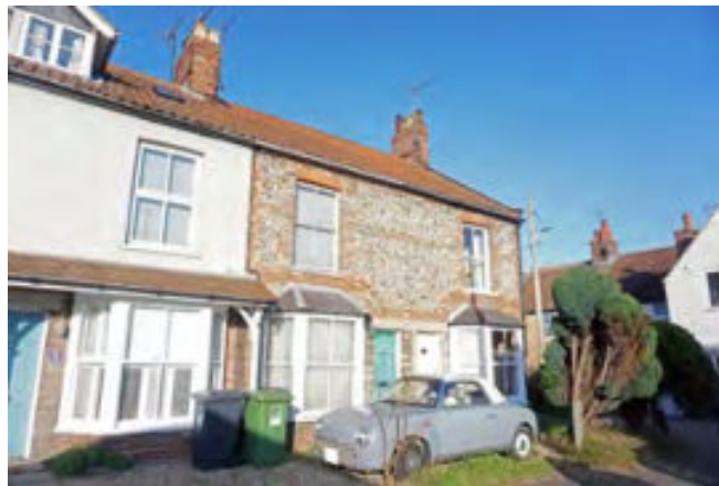
Cottages off Peacock Lane newly included within the Conservation Area boundary (area G on the plan)
