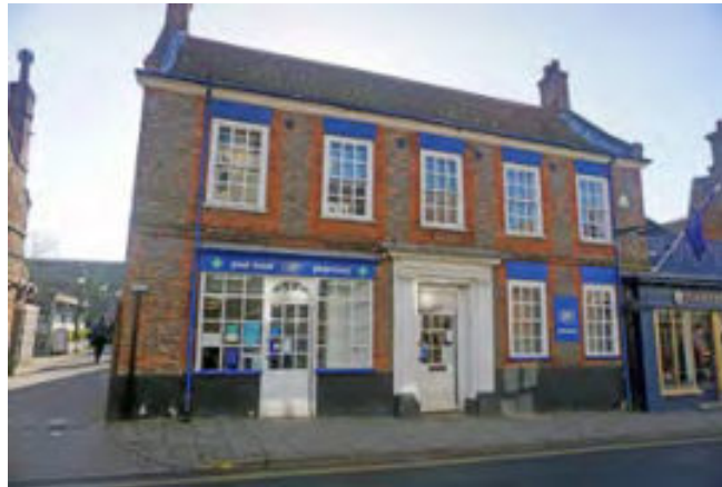
Red and brown brick to a Georgian building on the High Street, with sash windows, Classical doorcase and later inserted shop front. This building is likely to be amongst the earlier buildings to be reconstructed after the 1708 fire
