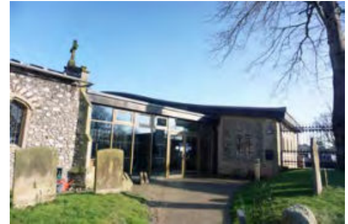
Extension to St. Andrew's Church
