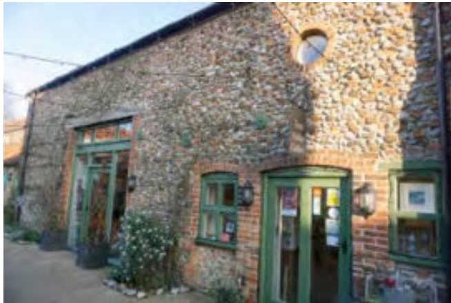
Converted outbuildings on Hooper's Yard
